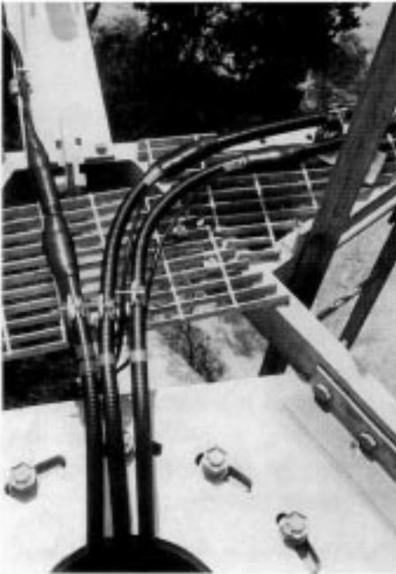
Figure 4: Top of a monopole showing angle adapters, standard hangers, butyl and vinyl tape weatherproofing, and ground kits on a monopole platform.
