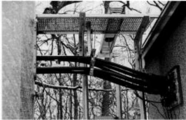
Figure 5: A cable bridge between a monopole and an equipment shelter. Accessories shown are entry port to the building, grounding bar, snap-in hangers, cable bridge support kit, and butyl and vinyl tape weatherproofing with ground kits.
