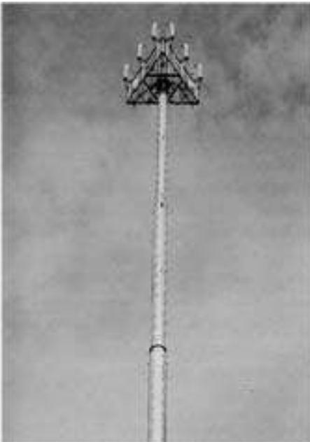
*Figure 1: A self-supporting monopole tower, such as this step-tapered version, is a typical choice for light cellular and PCS/PCN and light microwave applications.*
