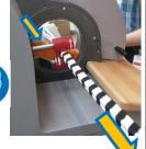
Cables shall be bundled using approved taping method.
