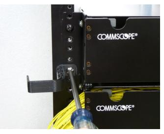
(3.) Connect Fiber Patch cords to module and run the cables out of chassis and over the accessory kit Vertical Cable Guide. Do this for both sides of the chassis.
