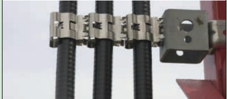
The anatomy of a stacking snap-in hanger
