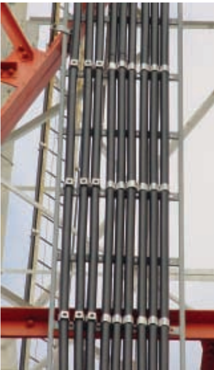
Existing cable runs can be remounted with stacking snap-in hangers to accept new runs on top.
