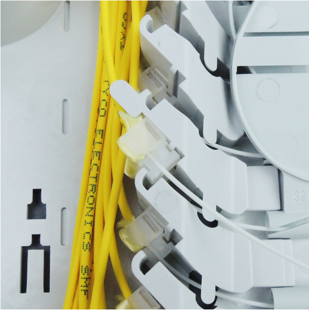
3.4 Slide the installed pigtail into the groove Note: you can stack up to 4 pigtails
