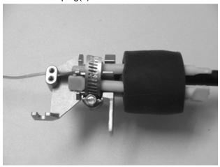
3.10 Protect the hose clamp and the termination with some layers of PVC tape.
