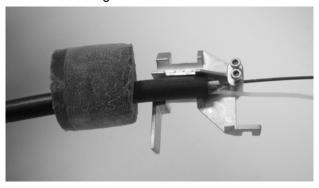
3.5 Fasten the screws to secure the strength member.
