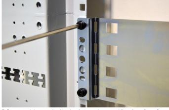
5.2. Mount the back plate, using an Allen key. Install further back plates "gapless".
