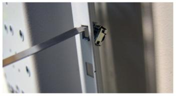
5.1. Determine the position of the back plate. Mount the cage nuts in the frame with the tool, as shown.
