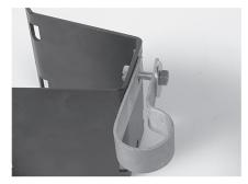
5. Fix the mounting bracket with the 2 rodclamps onto the rod.
