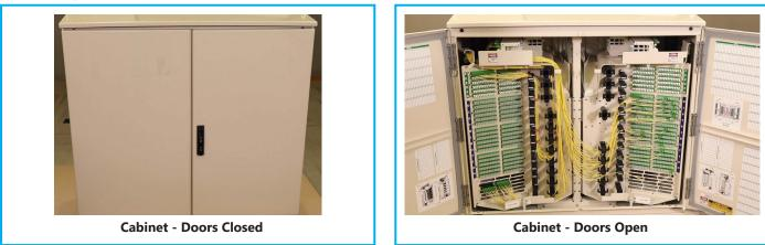
5.2 Inspect the internal parts of the FDH. The swing frames need to be in good condition.
