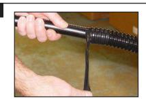
Remove electrical tape from the trunk cable and corrugated protection tube
