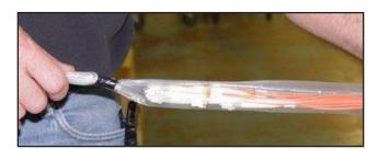
After you have pulled the fiber and power conductors remove electrical tape from the trunk cable and remove clear tube for access to all optical connectors.
